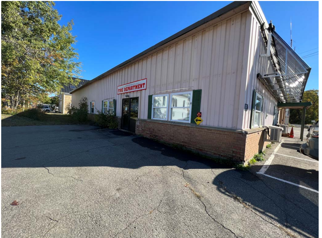
Fire Department Entrance
